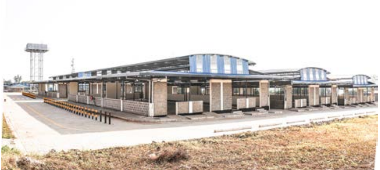
Uhuru Business Park Market Complex, Kisumu
