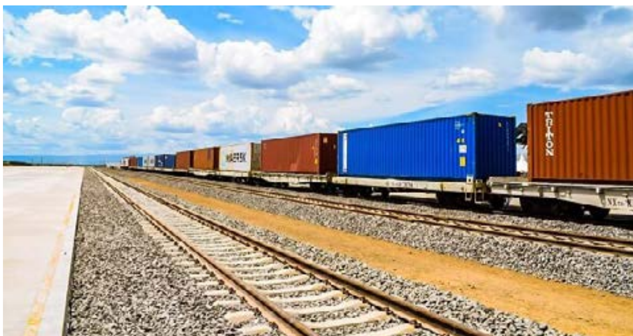
Naivasha Inland Container Depot
