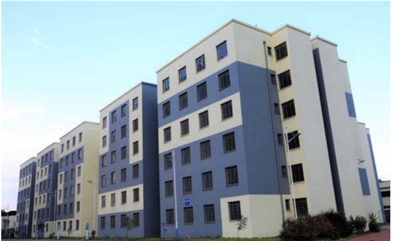
Parkroad Affordable Housing in Nairobi
