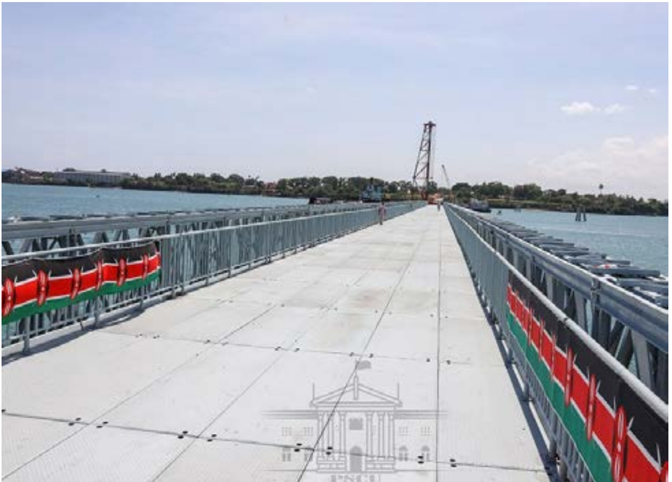
Liwatoni pedestrian floating Bridge, Mombasa
