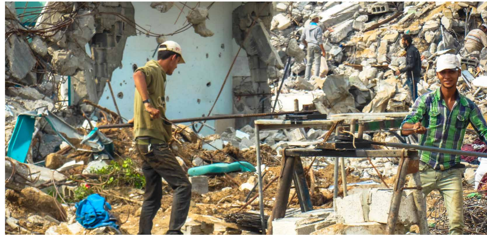
Photo 4.6. Construction workers re-using materials from destroyed buildings to reconstruct buildings in Gaza. Photo courtesy of UN-Habitat Palestine, 2015.
