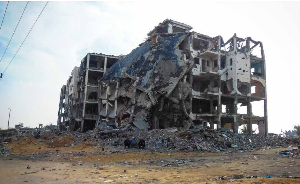
Photo 4.5. Destroyed housing blocks in Gaza. Photo courtesy of UN-Habitat Palestine, 2015.
