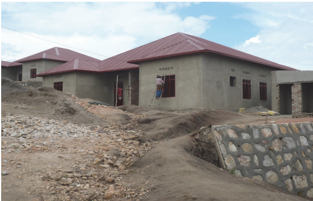
Figure 3.5. Block of four low-income housing units under construction
